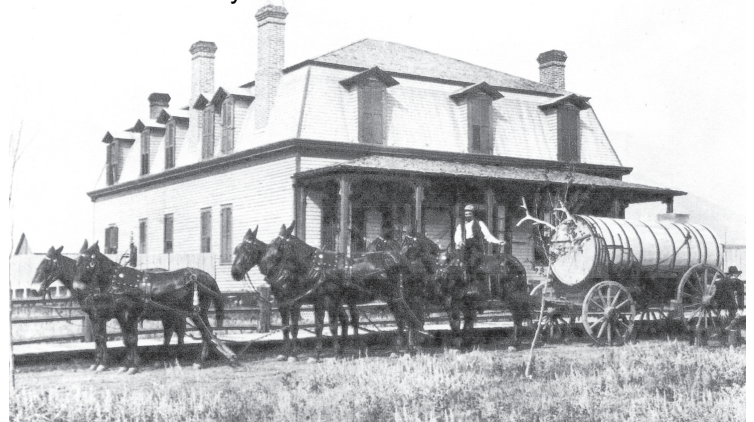
Water wagon in front of Commanding Officer's Quarters Photo: W. H. CULVER
