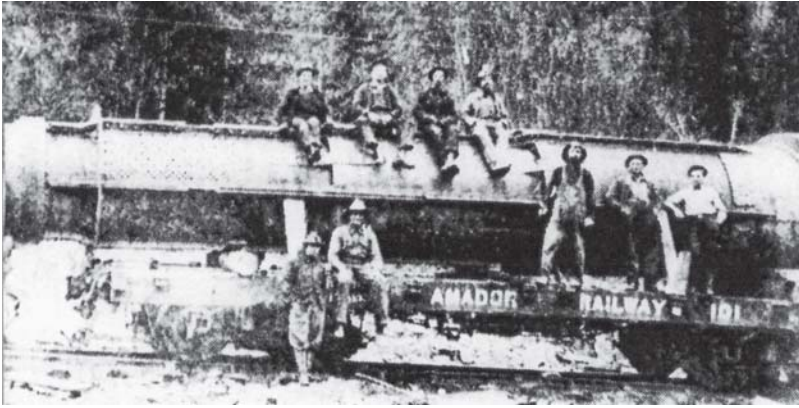
A huge 'Grizzly', used for cleaning ore, loaded on a flat car of the Amador Railway, for transportation to the 'Amador' mill that was under construction.
