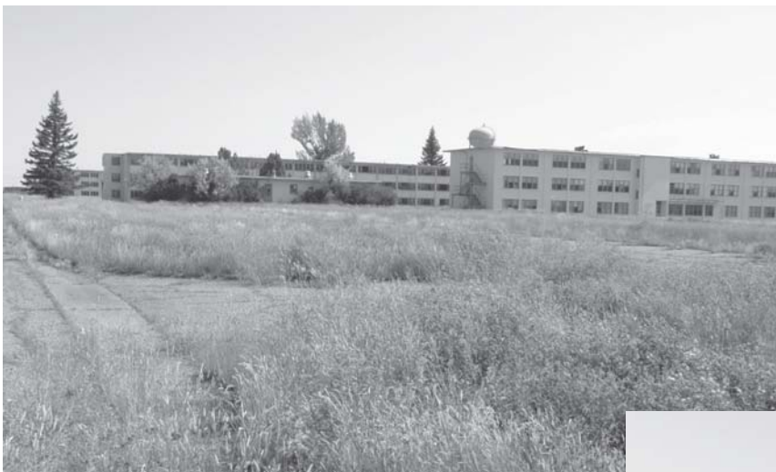
LEFT: Enlisted, single men's quarters (Closest to the airfield) All buildings are deserted.
