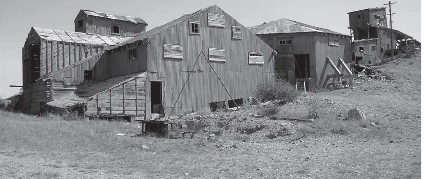
The mill at the 'Victoria' mine complex. All Photos: AUTHOR
