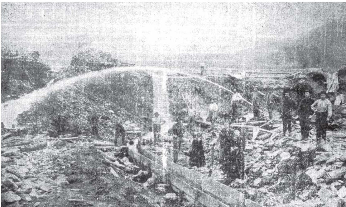
Hydraulic mining in Cedar Creek 1887. Louis Barrette is standing in the center of the three people on the right. The other two are the LaCasse brothers.
