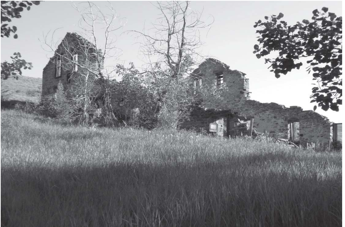
The east and west walls, all that remain, of the Elling - Morris mill, in Pony, built in 1883. It once had 20-stamps, each weighing 500 to 750 pounds, along with Frue vaners. It processed the ore from the 'Boss Tweed', 'Keystone' and 'Clipper' mines. TERRY HALDEN photo
