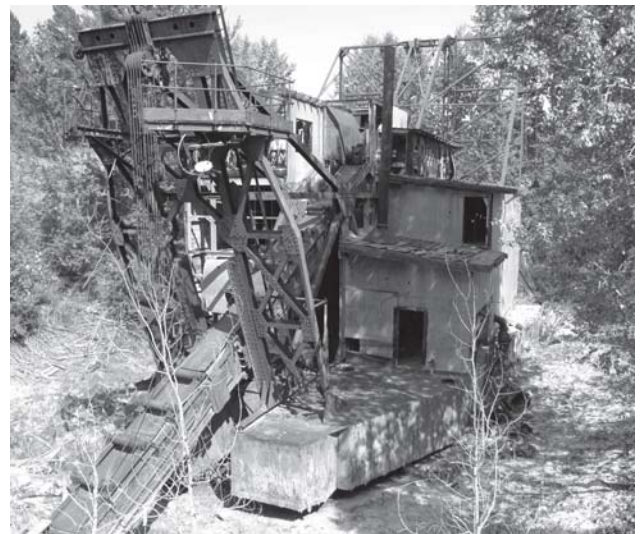
The remains of the dredge at Pioneer Creek, 2010. PHOTO: TERRY HALDEN
