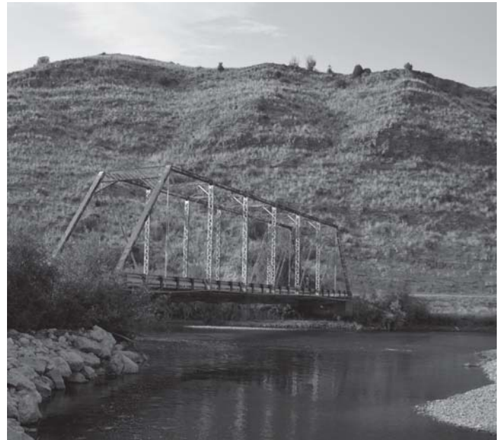
The Nixon bridge
