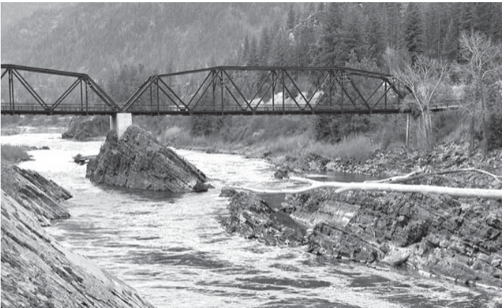
The bridge over Clark Fork river.
