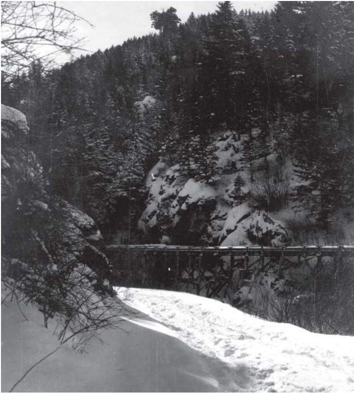
The old Cooper log flume in Bear Canyon that ran from the lumber camp near Bear Lake to Moffit Canyon. Photo courtesy GALLATIN HISTORY MUSEUM
