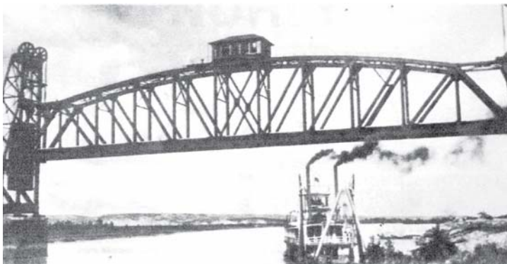
The southern span of the bridge in the raised position to let a paddle wheeler up-river.
