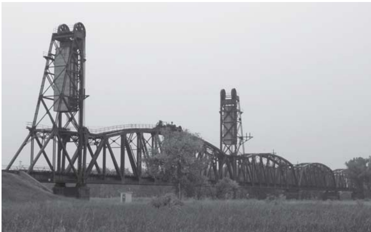
Another view of the bridge, lookin north-west.
