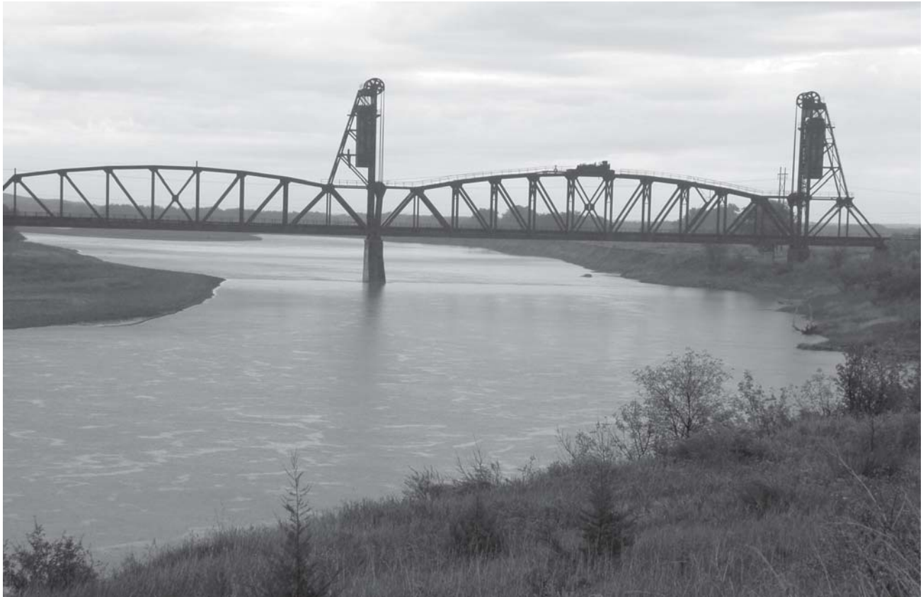
The Snowden/Nohly Bridge today, facing east
