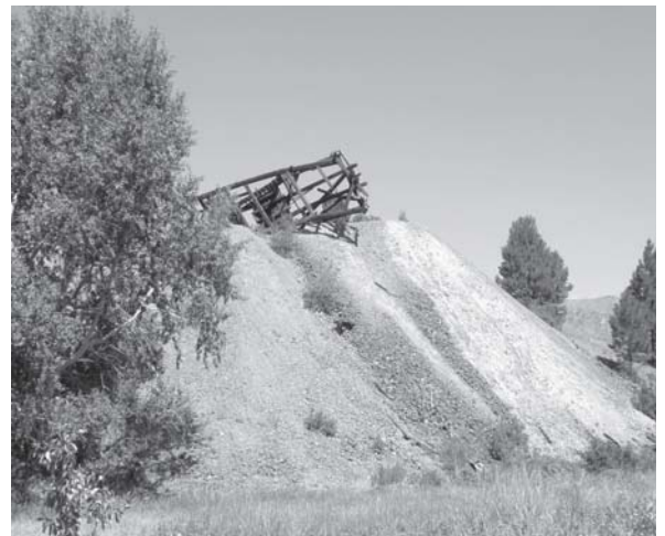
The collapsed head frame and tipple of the Economy Mining Company's 'John' mine on Mitchell Gulch. Photo: TERRY HALDEN
