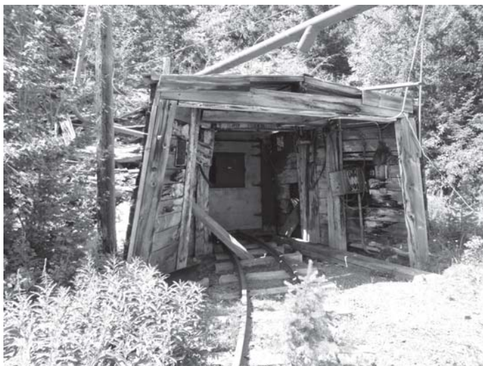
ABOVE: The adit to the No. 5 level of the Mouat mine.
