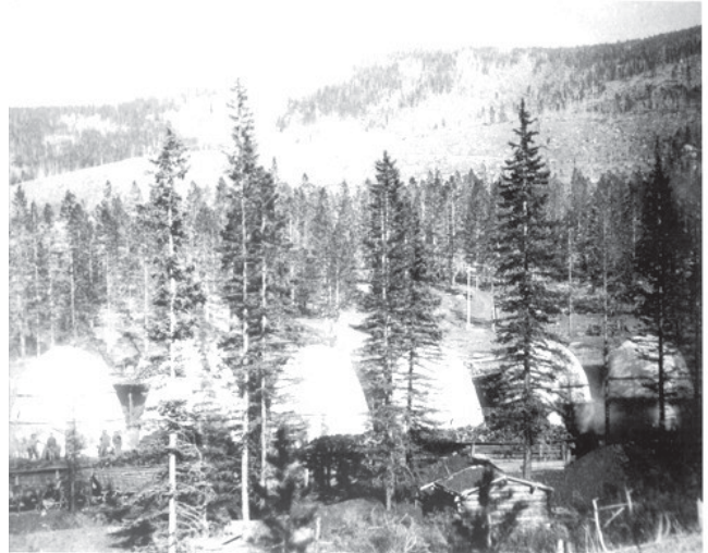
ABOVE: The kilns near Greenwood, on Trapper Creek after construction.
