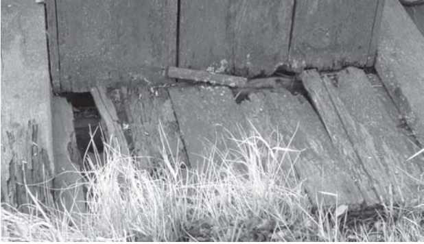
ABOVE: The rotten base of the well. RIGHT: Water-proofing the new base of the well.
