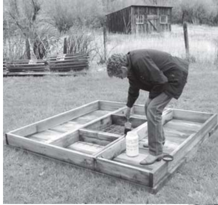
ABOVE: The rotten base of the well. RIGHT: Water-proofing the new base of the well.
