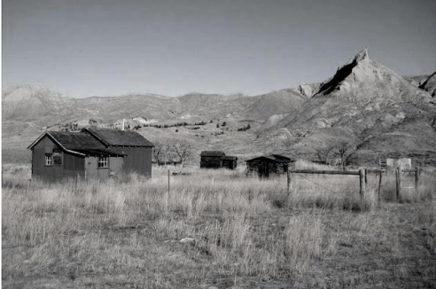
The Hagadone Homestead in 2008. BLM Photo
