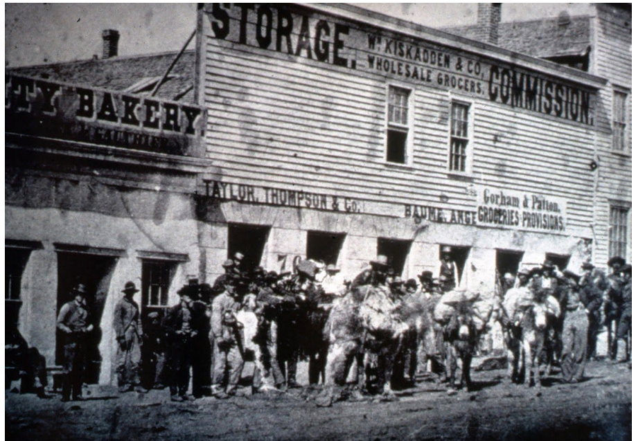
The Kiskadden Barn sports a tall false front and on the ground level, plaster scored to look like cut stone.
