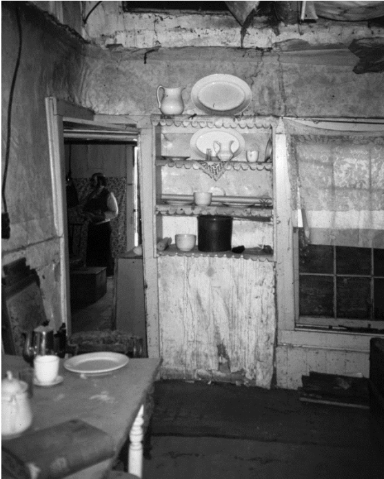
Muslin stretched smooth over log ceiling and walls, seen here in the McGovern Store, made interiors seem like finished rooms. Author Photo
