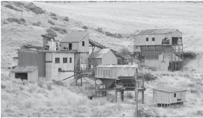
The Smith mine complex (Conveyor, coal processing plant, coal washery, scale house and tipples), today. Most of the buildings were rebuilt after a 1945 fire.
