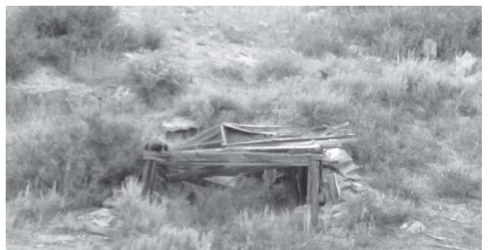
The collapsed Smith mine adit which had been constructed from dry laid sandstone with logs, boards or poles incorporated in the walls. LINDA DUTCHER photo
