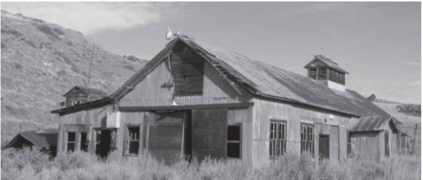
The Blacksmith and repair shop. It also included a coal analysis laboratory, electrical shop and offices.
