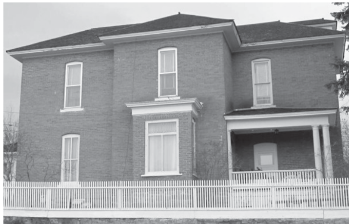
The hospital built by Dr. William H. Allen, physician for the Hope Mining Company, in 1887, is now a private residence.
