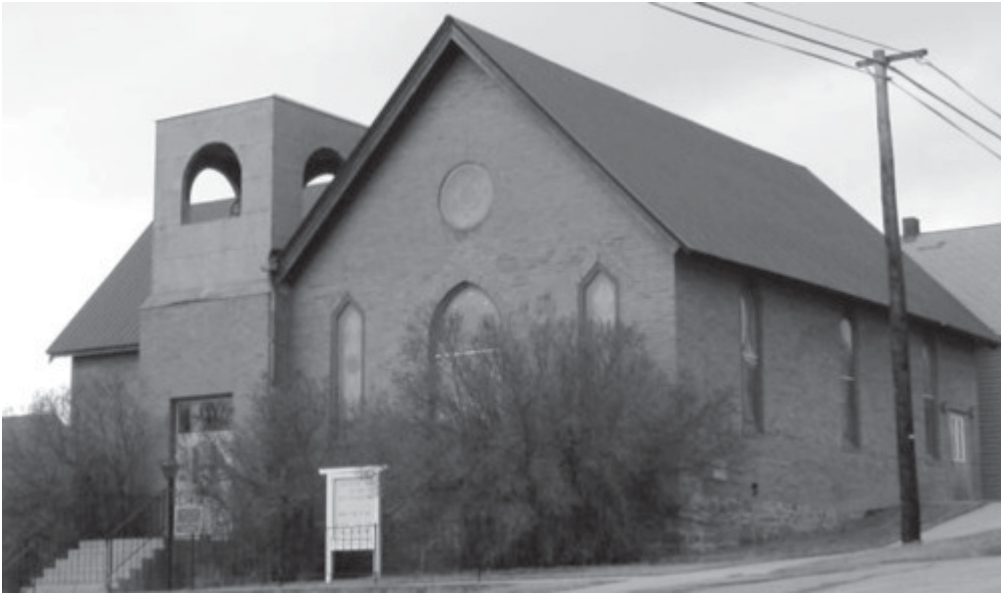
The cornerstone of St. Paul's Methodist Episcopal Church was laid in 1887. It is now owned by the Presbyterian Church.
