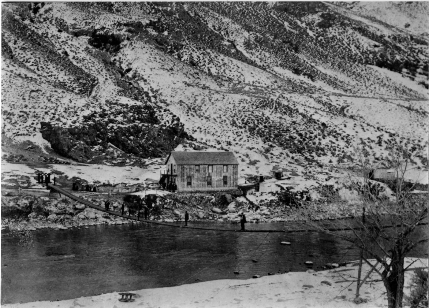
THE LaDUKE HOT SPRINGS SPA Ca 1903 WITH THE SWING BRIDGE
