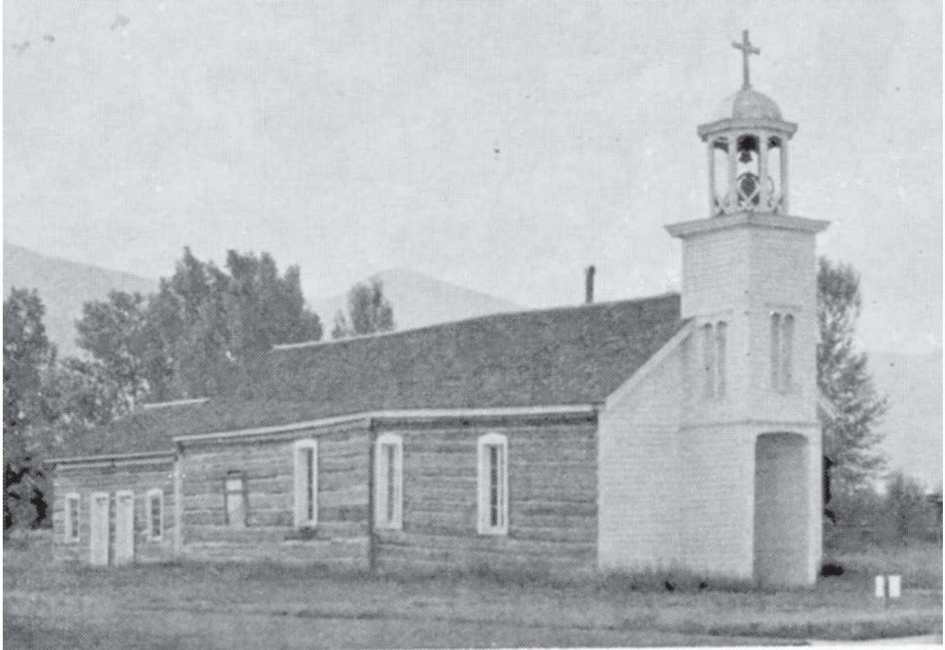
ST.MARY'S MISSION, AFTER IT WAS REBUILT.
