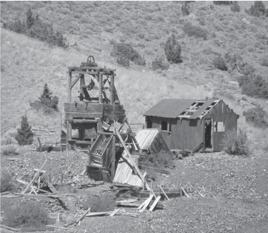
THE HEAD FRAME AND COMPRESSOR SHED AT THE 'MONTANA SILVER STAR' MINE, 2008.
