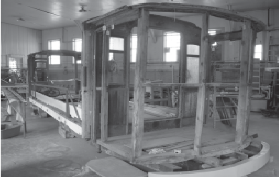
TROLLEY CAR No. 3 UNDER RE-CONSTRUCTION (Terry Halden photo)
