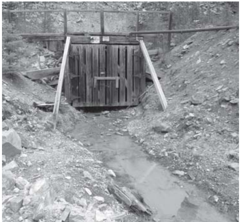
Although all work had ceased on the site, the culprit, the 'Gray Eagle' was still leaking its toxic waste. The stream in the original photo was orange in color.
